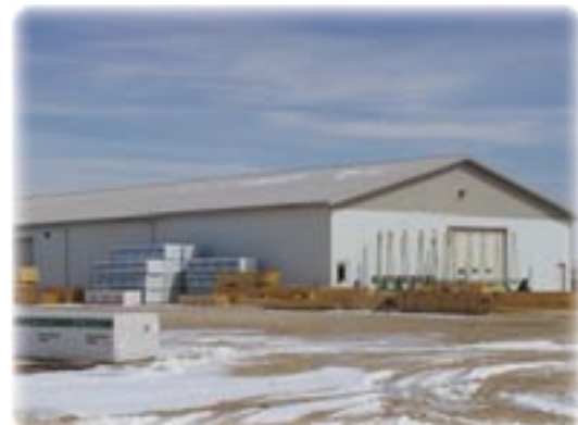
The truss manufacturing operation at the Prairie Blossom Hutterite Colony
