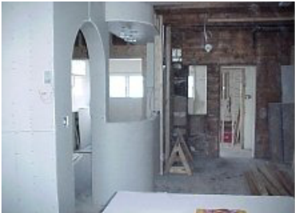
HOP house during renovation
